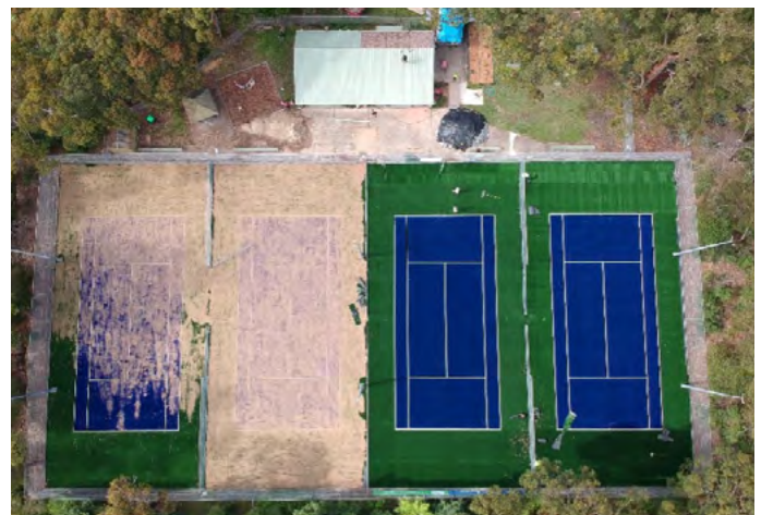
Figure 3: Aerial shot (Jan 2022) of the partially completed resurfaced tennis courts.
